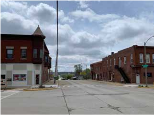
Existing street conditions at St. Paul Street and S. Spalding Street.
