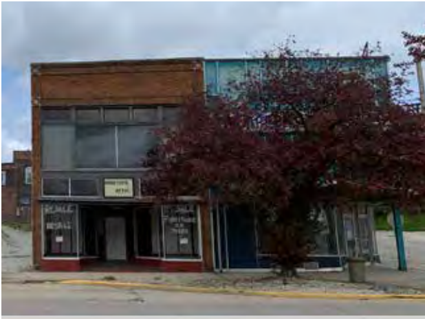
The existing St. Paul Street bump-outs.
